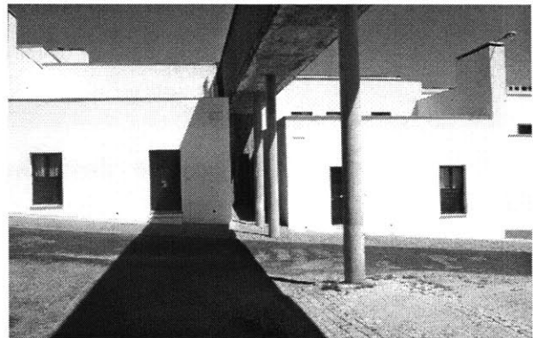
Figure 4.11 - Public housing and the service duct.
