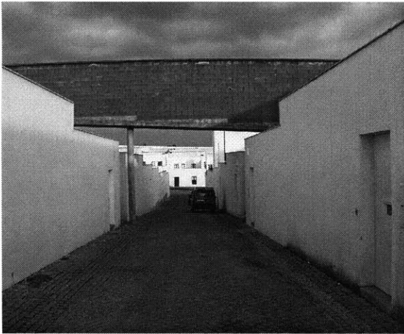
Figure 4.14 - The service duct passing over a pedestrian street.
